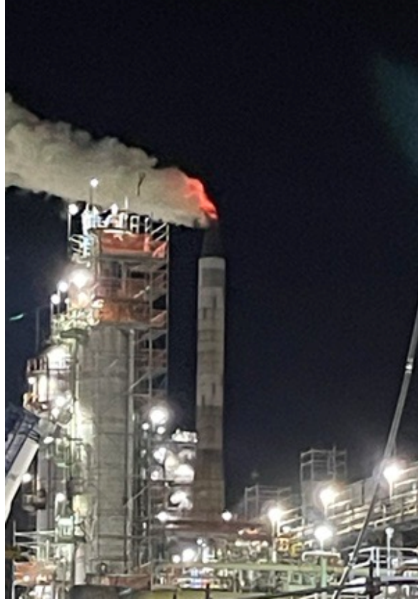
Figure 2: Thermal oxidizer experiencing low fire box O_2 during a high H_2S event.
